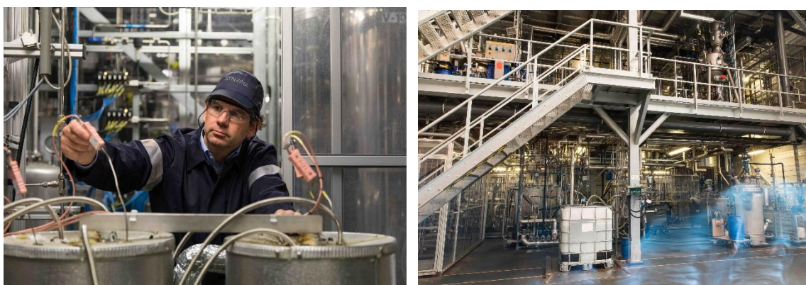
YXY® Technology Pilot plant in Geleen, The Netherlands
